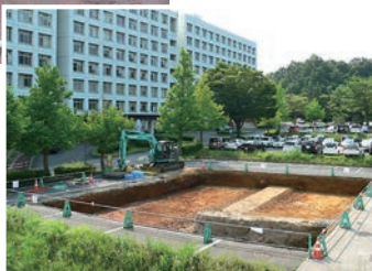
Decontamination measures (trenches drilling)
